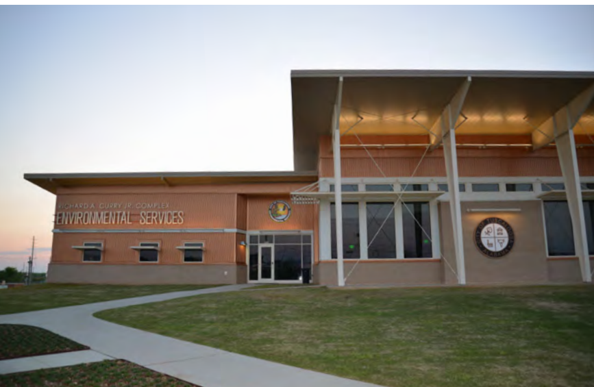
The new facility is now open and houses a state-of-the-art recycling center. (Photo by City of Tuscaloosa)
