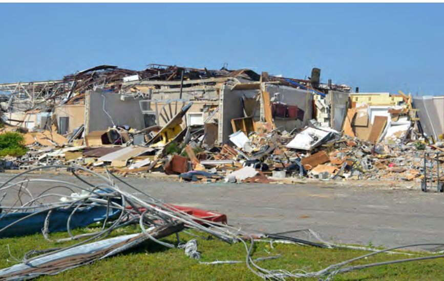
Tuscaloosa's Curry Building, which housed the City's emergency management division and environmental services, was completely destroyed on April 27, 2011. (Photos by Carrie Banks)
