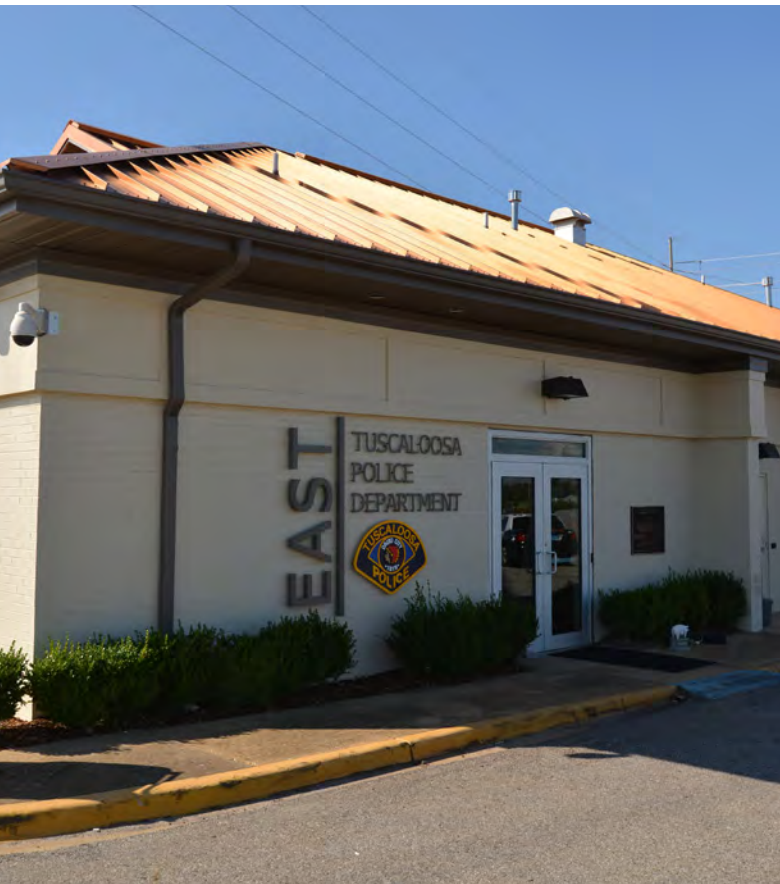
Tuscaloosa’s East Police Station was heavily damaged by the April 2011 tornado and a temporary unit was required (top photo). A new facility was built and is now open. (Top photo by Carrie Banks; bottom photo by City of Tuscaloosa)
